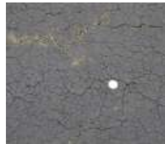
Spider cracks form rapidly in all seal coated surfaces.
